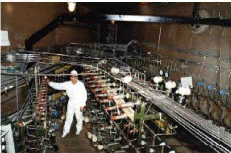
*Fire-retardant materials were applied to cables and wall openings at the Russian reactor in Smolensk. Should the cables catch fire, the retardant prevents fire from traveling along cables and damaging other systems, including those used to safely shut down a reactor.*
