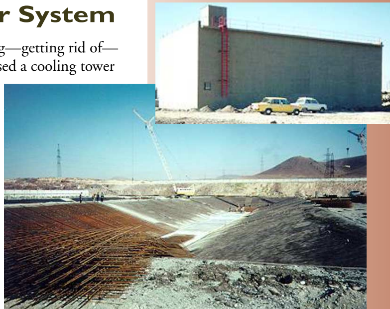
Three seismically hardened spray ponds will replace the cooling towers at the Armenia nuclear power plant. Pumps in pump houses (inset) will circulate cooling water between safety-related equipment in the plant and the spray pond.
