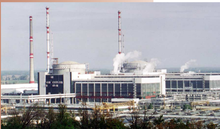
Kozloduy nuclear power plant, Units 5 and 6. The plant is implementing seismic upgrades, based on an assessment by U.S. and Bulgarian specialists.
