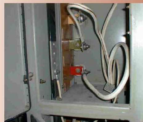
The infrared camera clearly shows hot spots in this electrical junction (top) that are not visible otherwise (bottom). The equipment is being used at the Kozloduy plant.
