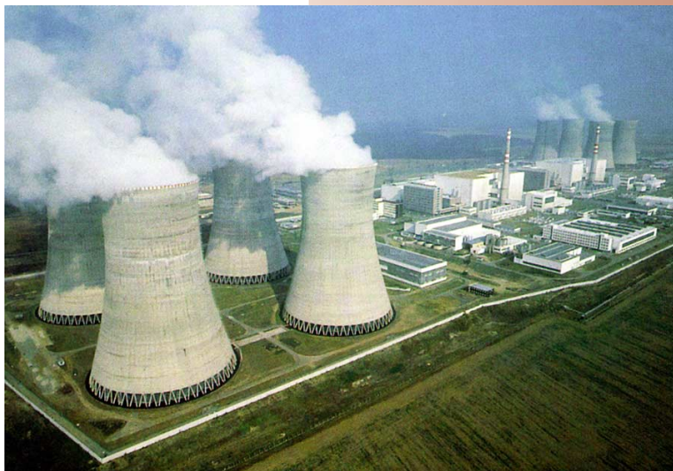
Dukovany nuclear power plant. With U.S. funding, Scientech experts will train Dukovany personnel in 1999 to use a risk advisory software program.
