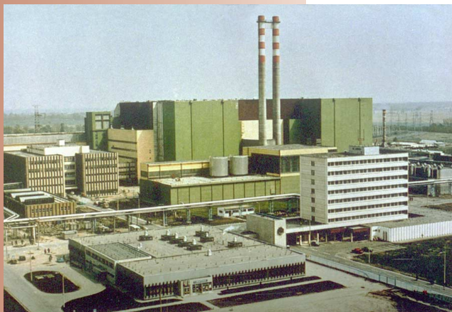
Paks nuclear power plant. Staff from the U.S. Department of Energy's Argonne and Pacific Northwest national laboratories have supported analyses of plant systems.
